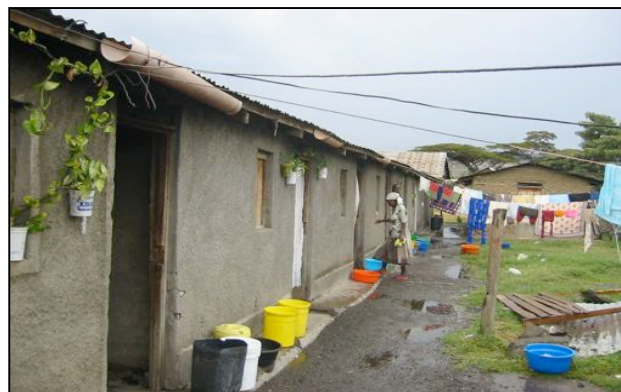
Upgraded housing in Nakuru. Very simple dwellings but note the impermeable walls, the step to prevent water penetration – and the plants show a pride in the dwelling!
